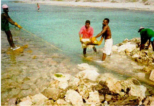
Figure 6. Placement of smaller rocks on top of Reef Ball breakwater.
