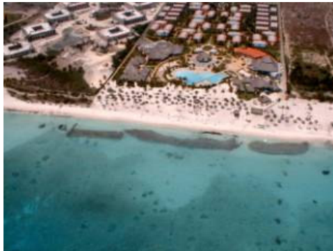
Figure 3. Three-Row Submerged Breakwater.
