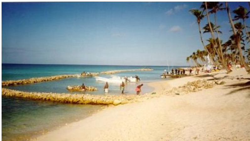
Figure7. Rock placement on top of Reef Ball breakwater and connected to shore.
