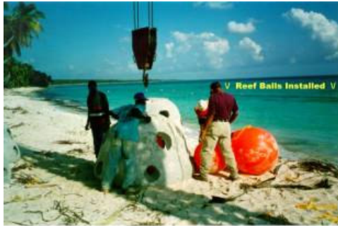
Figure 1. Individual Reef Ball™ Unit.
