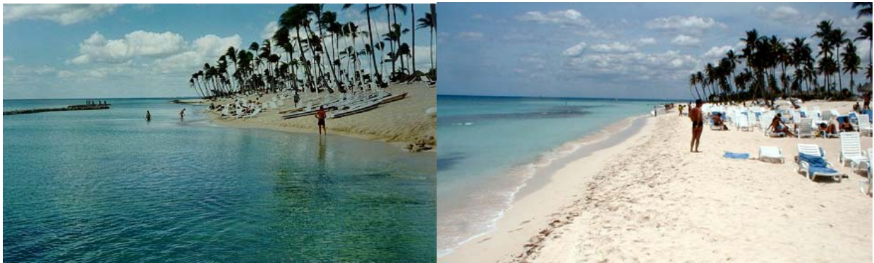
Figure 10. Increased Beach Width at Center Project - looking west.. February 1999 after small rocks added on top of breakwater (left), compared with April 2001 showing large natural accretion (right).
