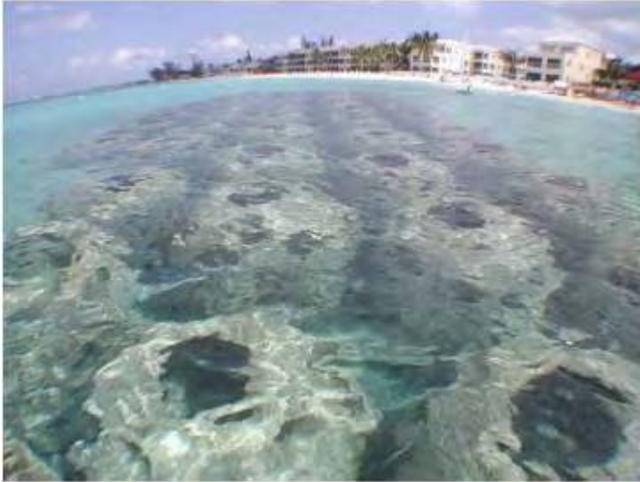
Figure 14. Grand Cayman Marriott Five-Row Reef Ball Submerged Breakwater
