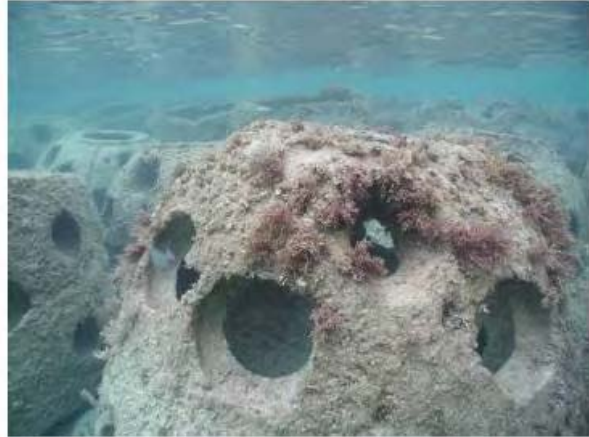
Figure 14. Grand Cayman Marriott Five-Row Reef Ball Submerged Breakwater
