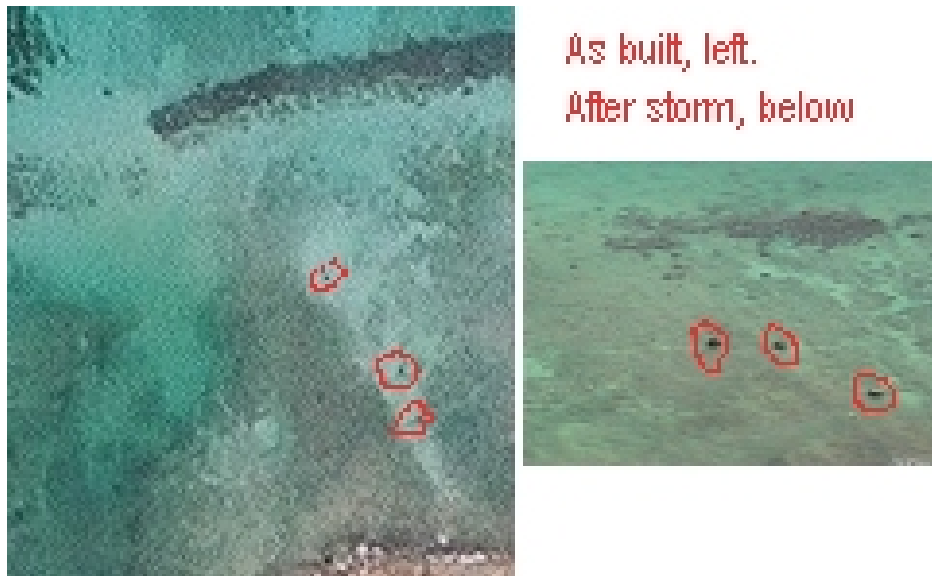
Figure 12. 3 Reef Ball Units Shoreward of Region D in the As-built Photograph on the Right, and Post-Hurricane Ivan Aerial Photograph on the Left. Note the 3 Reef Ball units shoreward of the breakwater in both photographs, and the displaced units in the breakwater after Hurricane Ivan.
