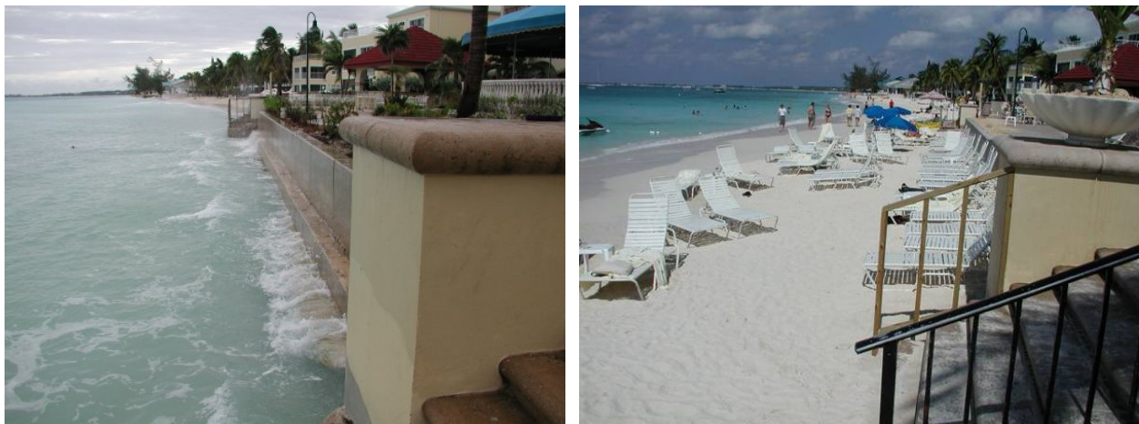
Figure 7. Before and After Breakwater Installation Photographs – View North October 2002 (left) and February 2003 (right)
