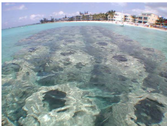
Figure 5. Grand Cayman Marriott Reef Ball Artificial Reef Submerged Breakwater - Above (left) and Underwater (right) Photographs.
