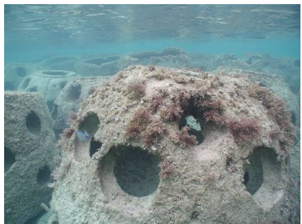
Figure 5. Grand Cayman Marriott Reef Ball Artificial Reef Submerged Breakwater - Above (left) and Underwater (right) Photographs.
