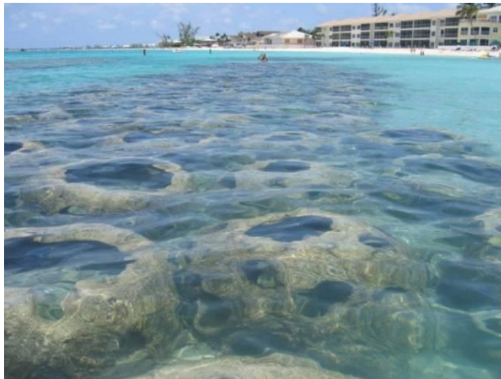
Figure 7. Reef Ball Breakwater after installation in Grand Cayman Island. (Photo courtesy of Lee Harris)
