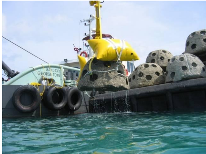
Figure 6. Reef Balls being deployed from a barge. (Photo courtesy of Lee Harris)
