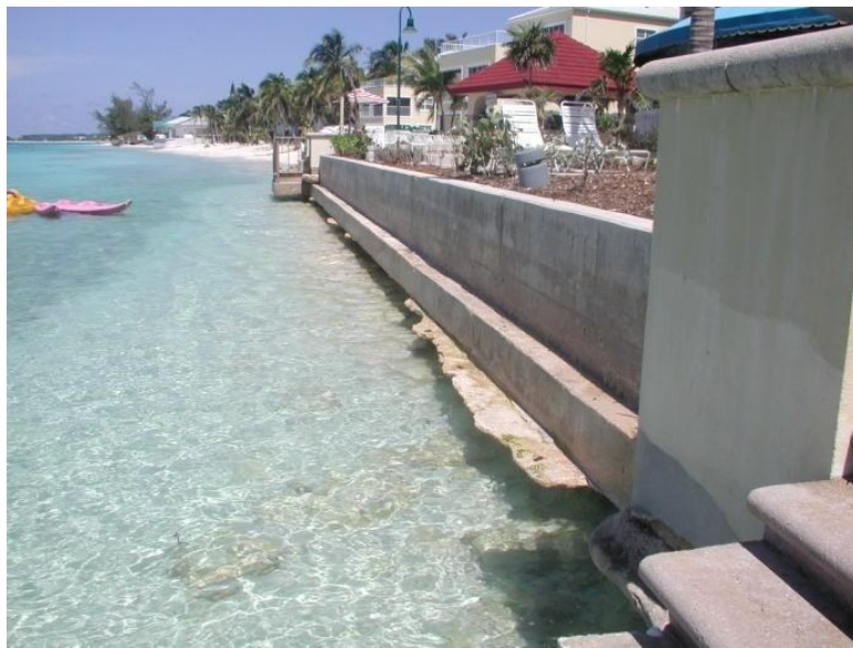
Figure 10. View looking to the North at Marriott seawall in 10/02. (Photo Courtesy of Lee Harris)
